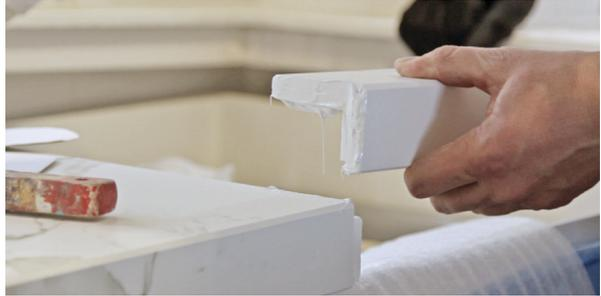
**1)** Clean the area, removing all dirt and dust. Before adhesion, It is advisable to place masking tape on both sides of the join to keep your work clean.
