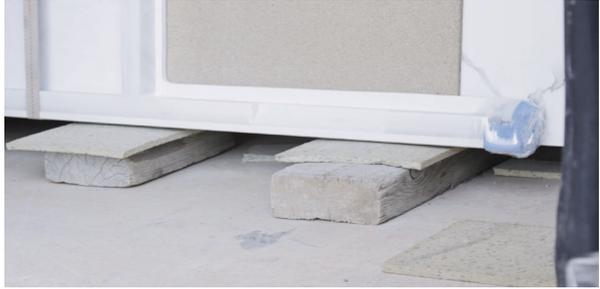
B) Place the product on both sides of the trestle, balancing out the load and ensuring that the pieces fit snugly into the frame.
