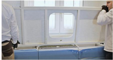
3) Review the supports of the units where the worktop will be attached. They must rest properly on the floor, and be solid and
